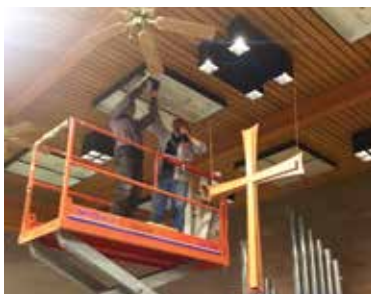
Installing energy efficient lighting in Hosanna's sanctuary.
